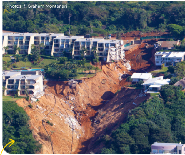
Devastating landslide damage at Umdloti, Durban, following the 2022 KwaZulu-Natal floods, which destroyed sections of residential buildings and surrounding infrastructure.
